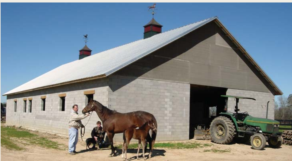
As interest in the dry stack method grows, the use of VOBB concrete blocks for other types of construction projects increases as well. Rocky Landry, owner of this horse barn in Iberia Parish, chose concrete block after a long search for a product that would remain cool, even in Louisiana’s humid climate.
