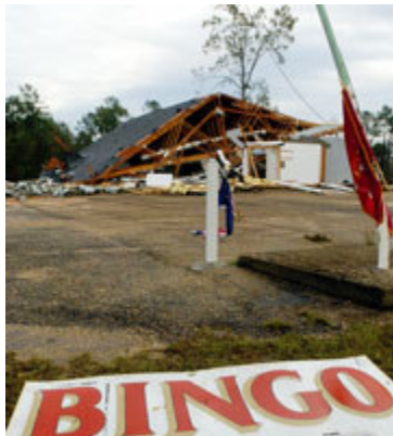
A tornado hit VFW Post 9122 in Mendenhall, Miss.
